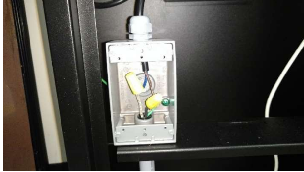
Figure 11 - Connect Incoming AC Power per local code and NEC
