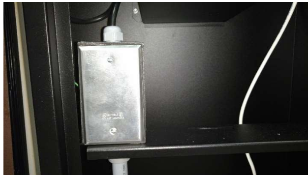
Figure 12 - AC Connection Complete, Junction Box Sealed
