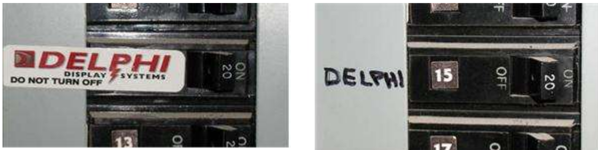
Figure 13 - Examples of Properly Labeled Circuit Breaker
