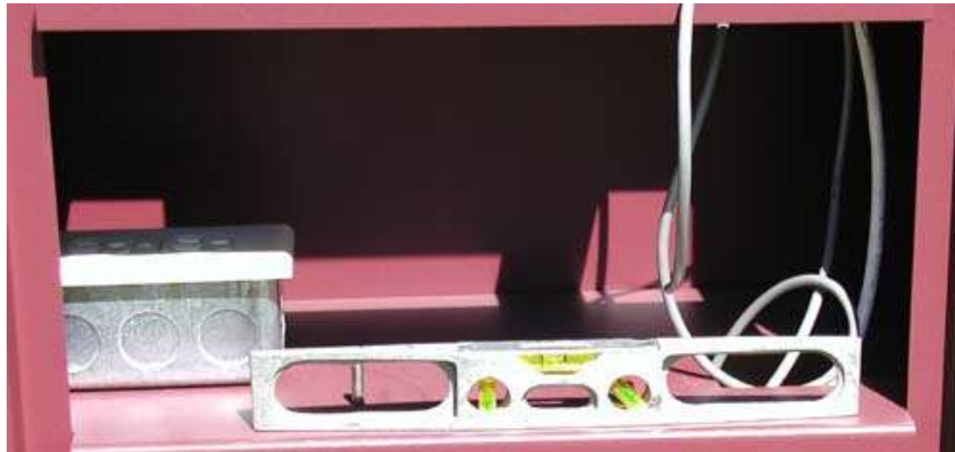
Figure 7 - Verify Post is Level
