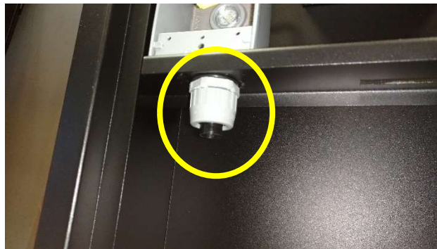
Figure 9 - Lower Nipple for AC Electrical Connection
