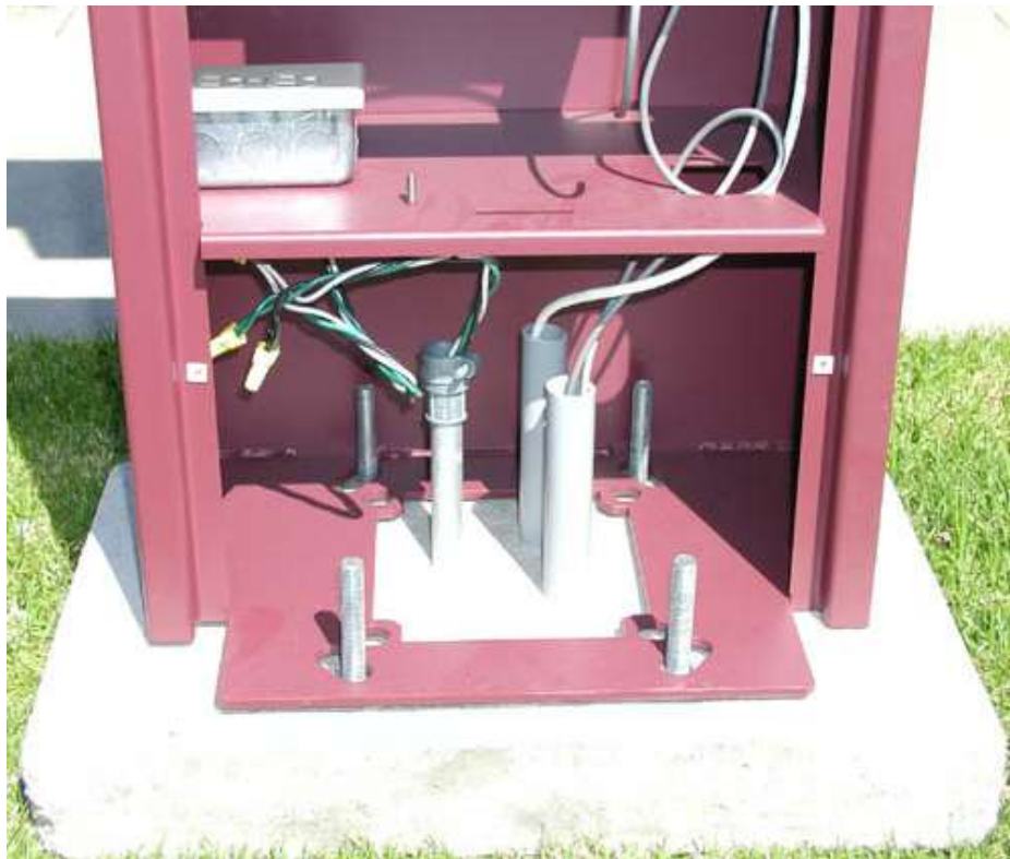
Figure 5 - Setting the Post on the Footing
