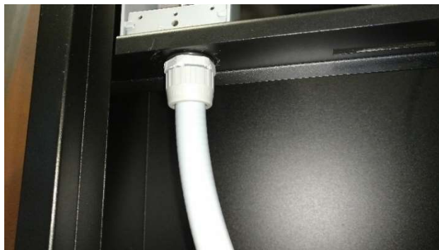
Figure 10 - Incoming AC Electrical Routed Into Junction Box
